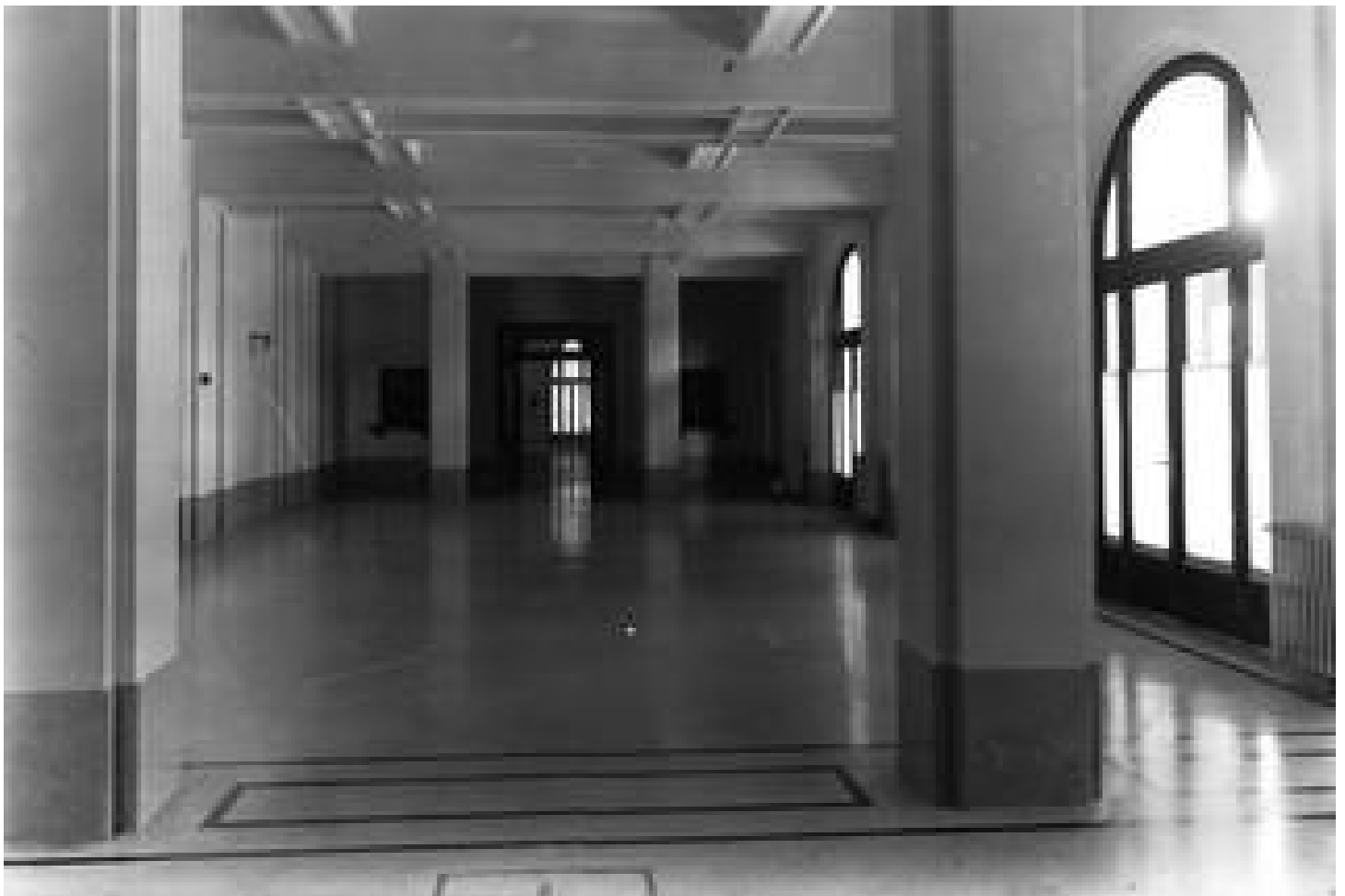
HALL PRINCIPAL -BIBLIOTECA-
